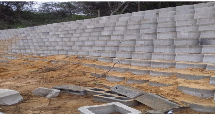
Top part of the Retaining Wall Completed
