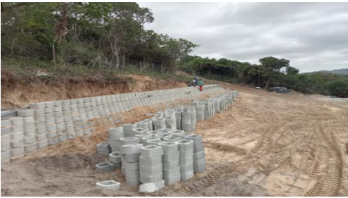
Retaining Wall Half Way to Completion
